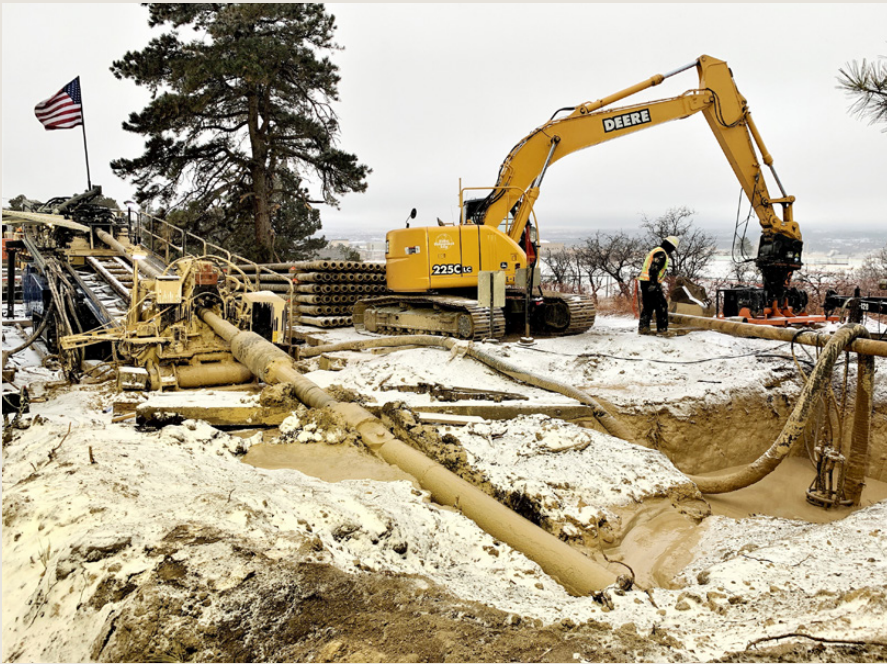
Figure 1. Completion of 10-inch HDPE DR 7.3 pipe installation
