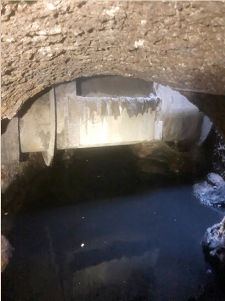
Interior Image 27-inch Dia Pipe Through 48-inch Dia Pipe Manhole Structure
