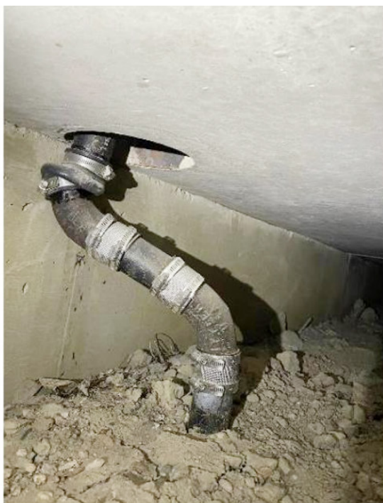
Figure 6. Yet Another Challenge to Overcome: Hand Tunneling to the Cleanouts While Ensuring Ventilation and Worker Safety in the Confined Spaces
