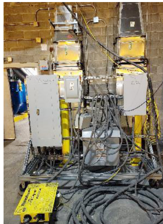
Figure 7. C&L Needed to Make Its Own Power Distribution Unit (PDU) to Accommodate Various Tool Requirements
