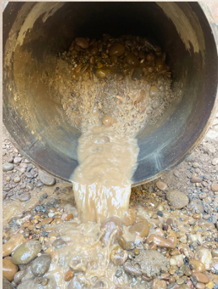
Figure 8. Soil and ground water encountered during pipe ramming operations
