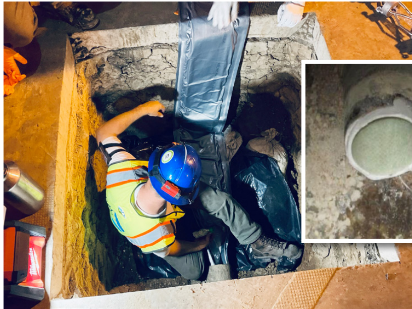
Figure 2. Installation Crew Uses Its UV-Light Cured CIPP System in the 2012 Job to Perform High-Quality CIPP Pipe Lining Installations from Excavation to Excavation in Slab-on-Grade
