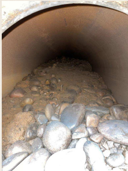
Figure 8. Soil and ground water encountered during pipe ramming operations
