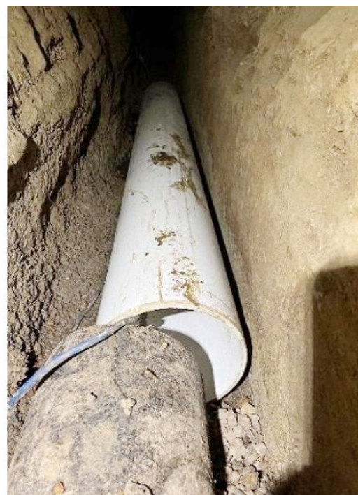
Figure 6. Yet Another Challenge to Overcome: Hand Tunneling to the Cleanouts While Ensuring Ventilation and Worker Safety in the Confined Spaces
