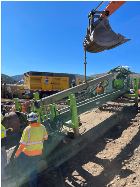
Desired 12 degree entry angle was met by adjusting independent hydraulic legs
