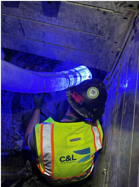
Figure 2. Installation Crew Uses Its UV-Light Cured CIPP System in the 2012 Job to Perform High-Quality CIPP Pipe Lining Installations from Excavation to Excavation in Slab-on-Grade
