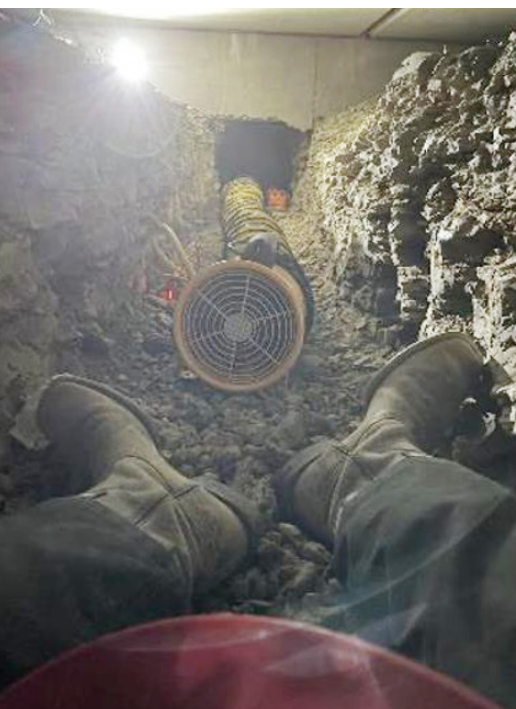
Figure 6. Yet Another Challenge to Overcome: Hand Tunneling to the Cleanouts While Ensuring Ventilation and Worker Safety in the Confined Spaces
