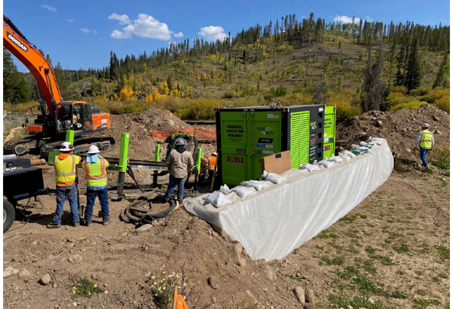
Drilling needed to go 240 feet through cobbles before hitting bedrock
