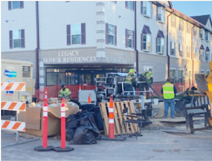
Excavation & CIPP Installation at Legacy Senior Residences
