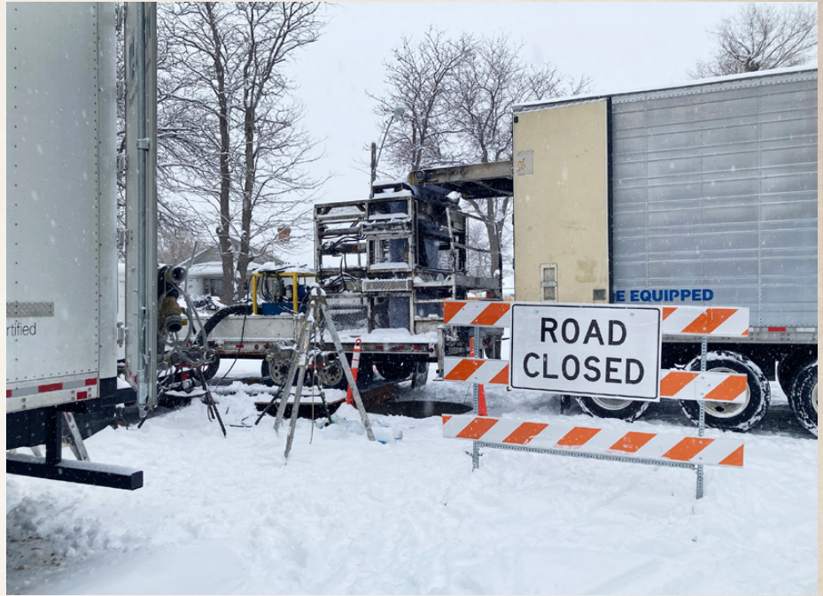
-5F Installation and -30F Cure Evening - cold snowy weather extended CIPP cure times
