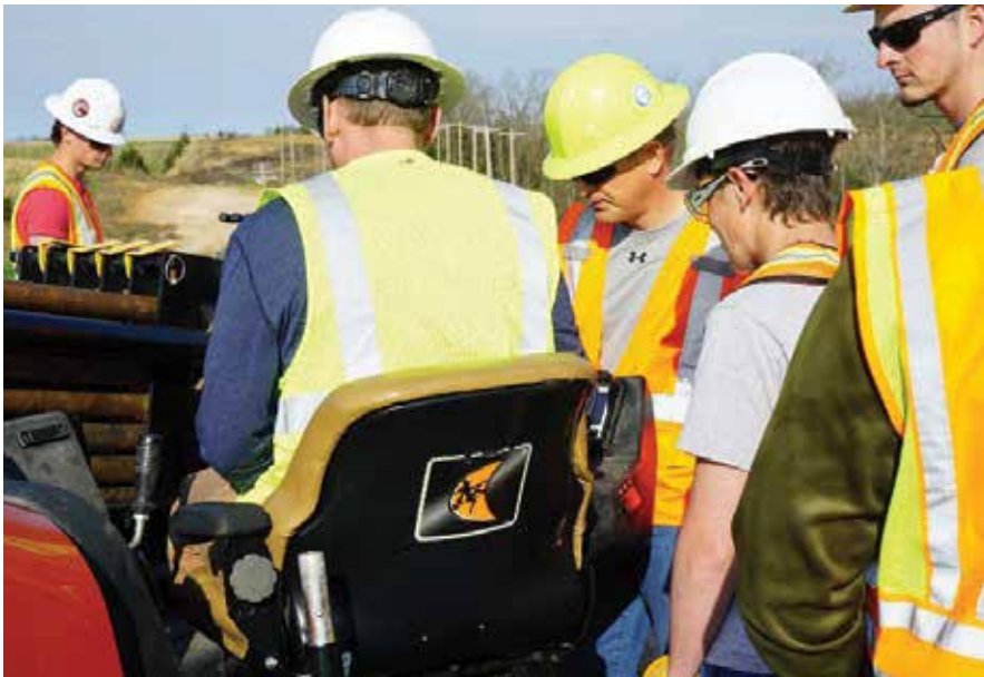
Figure 5. The Utility Systems Technician Program is focused towards hands-on instruction for students that are interested in joining the underground construction industry, allowing them to make an immediate impact in the field upon graduation.
