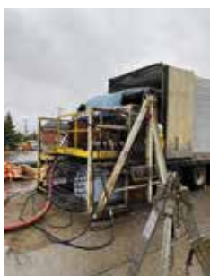
Figure 6: Liner 6104 – typical air inversion install
