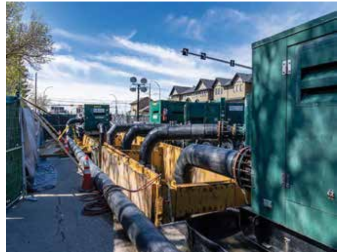
Figure 2: Bypass installation at main bypass pit
