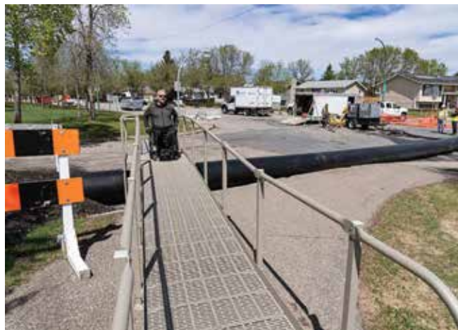
Figure 8: Wheelchair access ramp during construction
