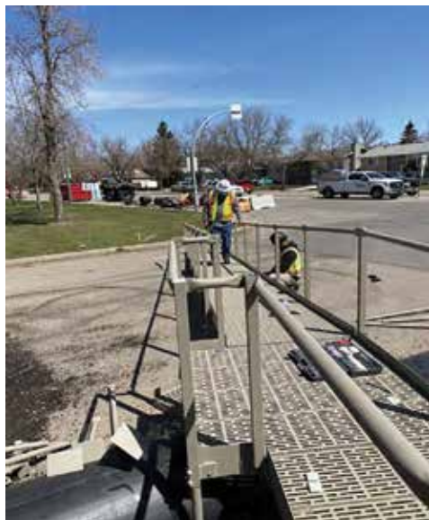
Figure 8: Wheelchair access ramp during construction
