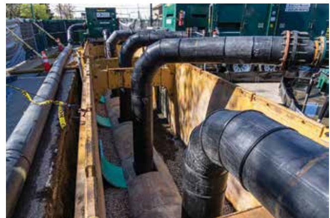
Figure 3: Bypass suction cored into pipe at main bypass pit
