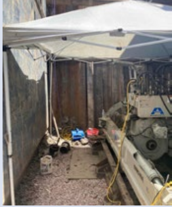
Before the machine can be set up, Morty and crew always make sure the bore pit starts out on line and grade. This Akkerman 240 GBM has it made in the shade
