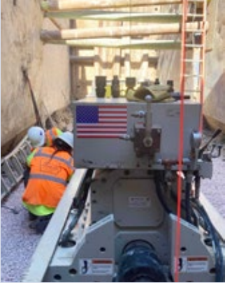
Before the machine can be set up, Morty and crew always make sure the bore pit starts out on line and grade. This Akkerman 240 GBM has it made in the shade
