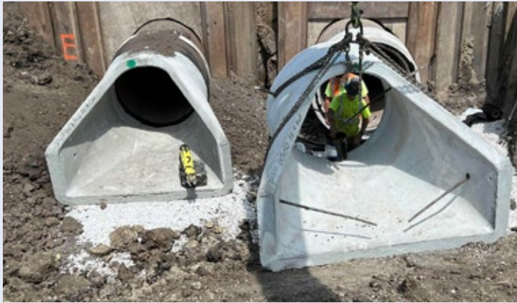
Twin 60-inch tunnels installed to replace a structurally deficient box culvert
