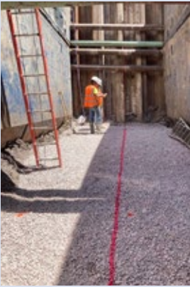
Before the machine can be set up, Morty and crew always make sure the bore pit starts out on line and grade. This Akkerman 240 GBM has it made in the shade
