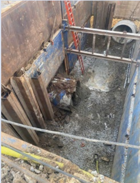
In order to make this project work, multiple tunnels shared one shaft, which had to be angled to accommodate both purposes, and allowing a receiving shaft to be the launch shaft for the next drive
