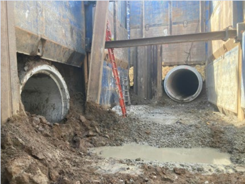
In order to make this project work, multiple tunnels shared one shaft, which had to be angled to accommodate both purposes, and allowing a receiving shaft to be the launch shaft for the next drive
