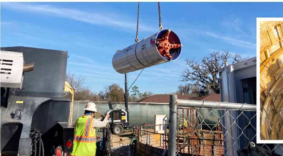
Lowering the MTBM into jacking shaft MH-T12 on Talton St.
