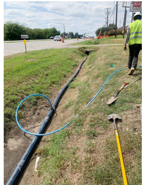
Temporary By-Pass Water Line
