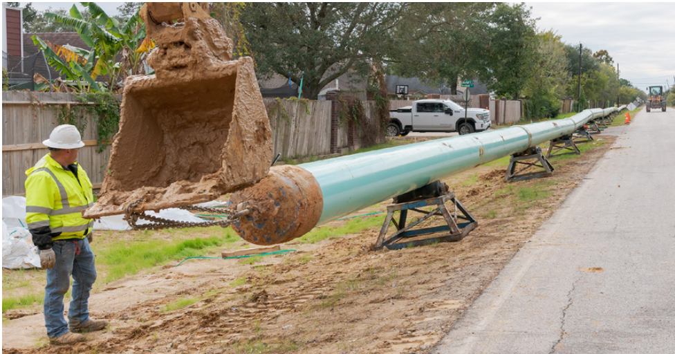
Pipe string is assembled during pullback
