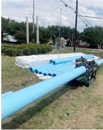
Fusible PVC® Pipe Being Fused
