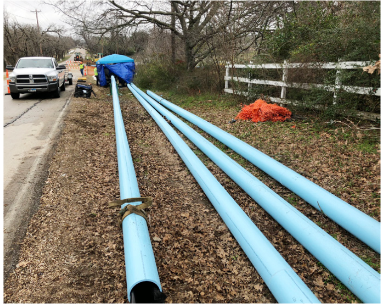
Joint fusing and pipe staging area. Sticks of PVC are joined to full run length prior to the day of the burst, stored conveniently out of the way near the insertion point
