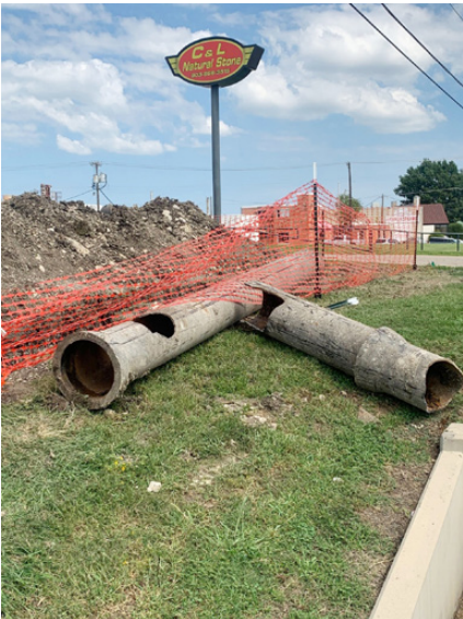
Original Cast Iron Pipe
