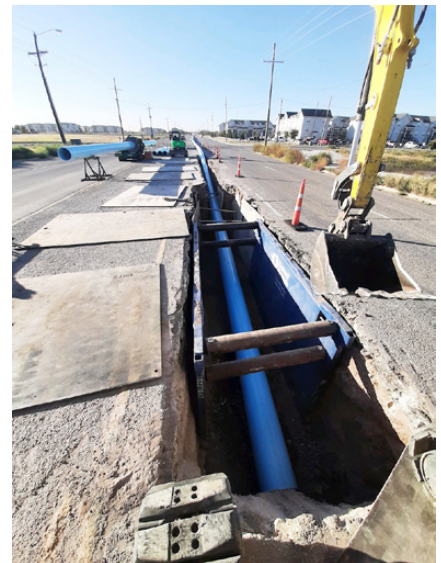
Average slipline pull lengths of 1800 to 2000 feet were achieved by the Contractor
