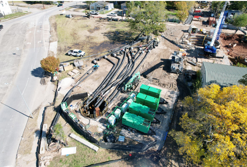
Maintaining road access was no small feat for this massive project
