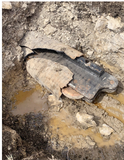
Static Pipe Bursting Head / Cutter
