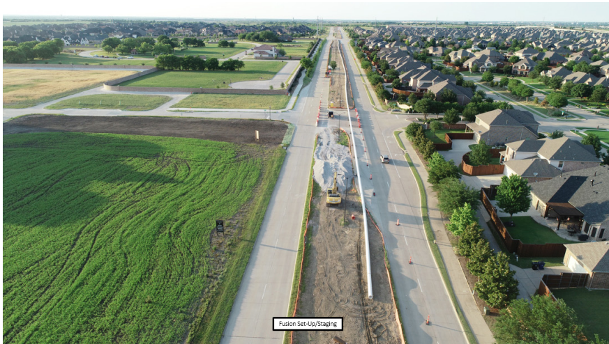
Figure 3 - Fused Pipe String
