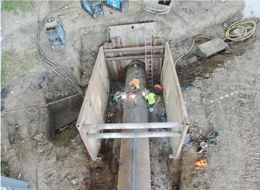
During the Conductor Barrel process, a casing is rammed in place at a predetermined angle. That casing serves several purposes including helping contain drilling fluid and allowing drilling to begin in optimum soil conditions
