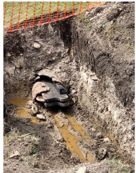
Static Pipe Bursting Head / Cutter
