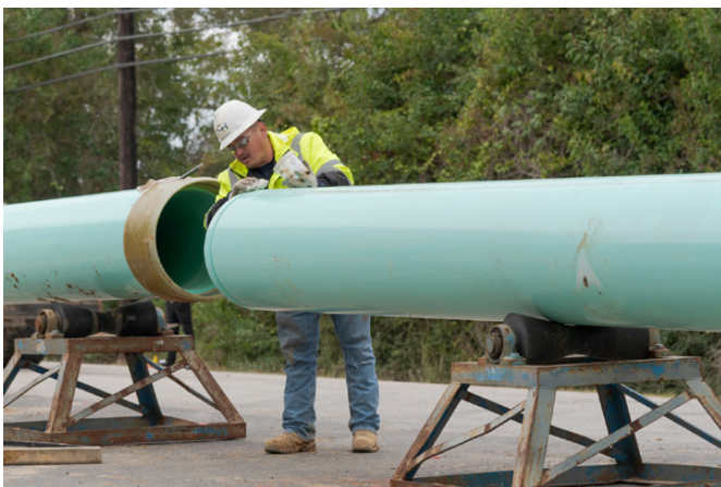
Speed and ease of the coupling system significantly reduces time and manpower
