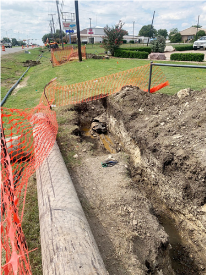
Congested narrow ROW. Pipe bursting reduced impacts to adjacent properties
