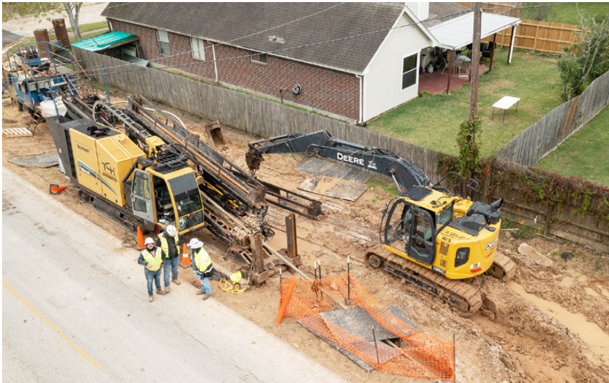
HDD offers minimal disruption to surface structures
