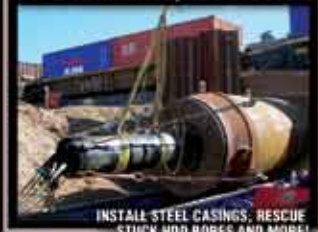
PIPE RAMMING/HDD ASSIST
