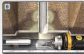
Grout collar stops infiltration
