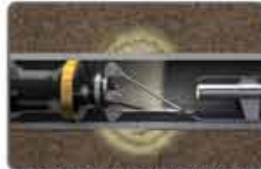
Grout collar stops infiltration
