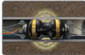
Chemical grout injected into soil
