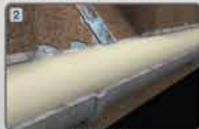
Liner installed
