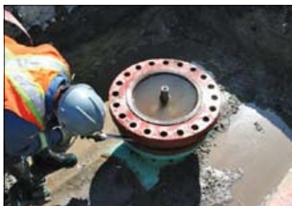
Figure 4. Line-stop completion plug
